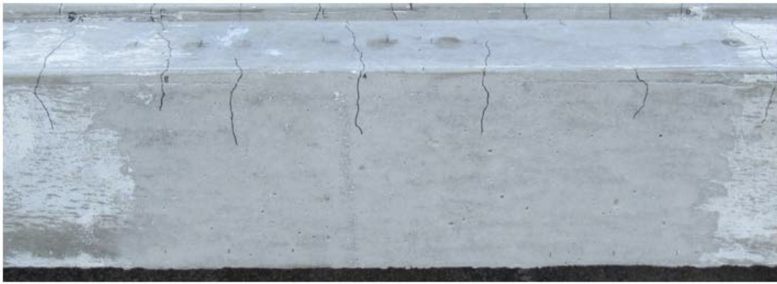
FIGURE 3.9 Flexural cracks
