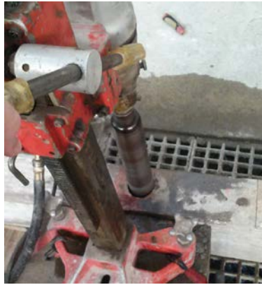
FIGURE 3.14 Coring process
