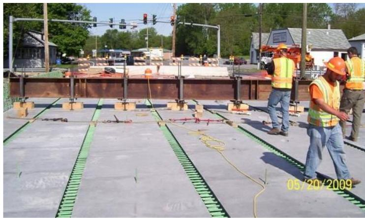
Figure 2.5 NYSDOT Bulb-Tee Girders with Shear Pocket Ready for UHPC Pour
