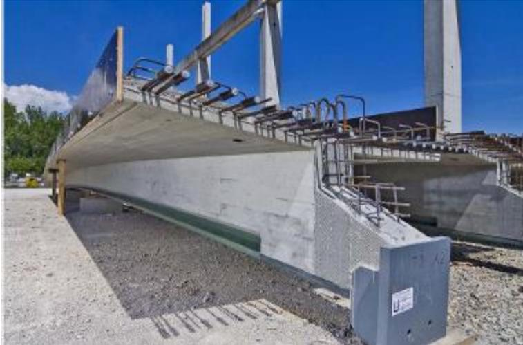
Figure 2.18 Prefabricated VFT Girder
