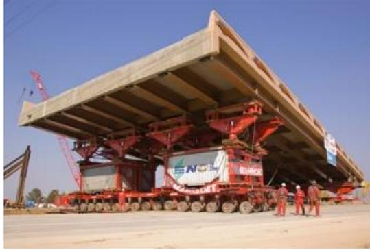
Figure 2.13 Bridge Span Being Moved with SPMTs
