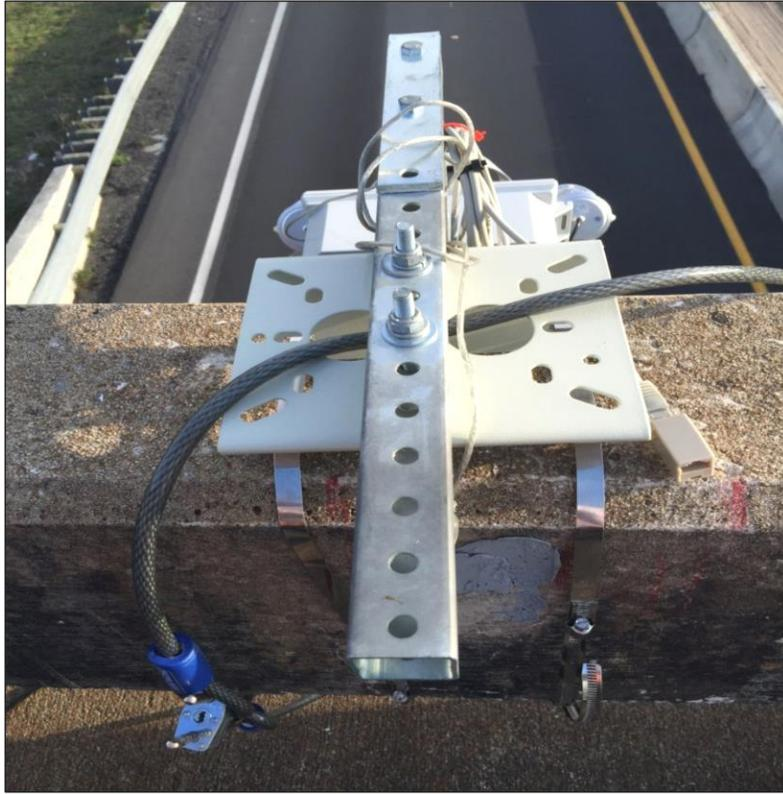
**Figure Error! No text of specified style in document.-7: Bracket Connection to Overpass**
