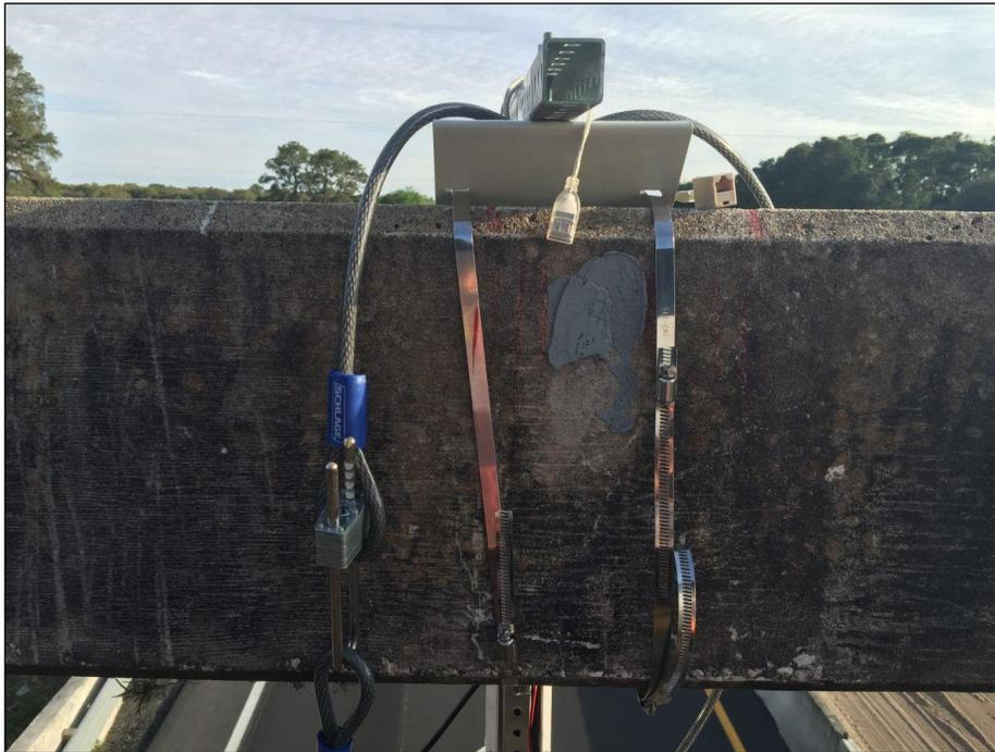
**Figure Error! No text of specified style in document.-8: Bracket Strapped to Overpass**
