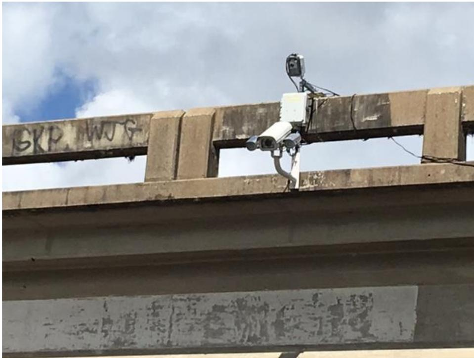
**Figure 4-8: Bracket Close-up Showing Sensor, Camera, and Processor**
