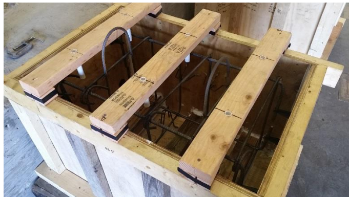
Figure 3.22. Formwork for Mustafa test specimens.
