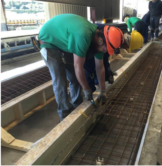
Figure 3.14. Formwork, welded-wire fabric, and prestressing
