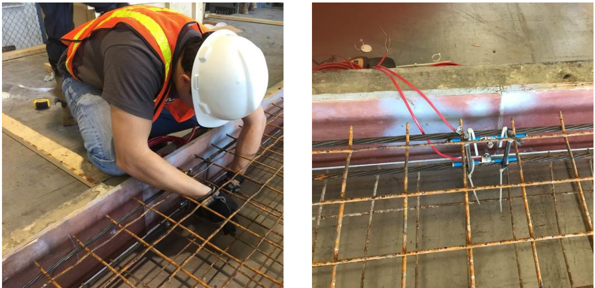
Figure 3.20. Installing vibrating-wire strain gages at midspan next to prestressing strands
