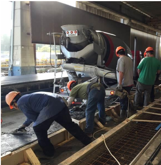
Figure 3.15. Placing concrete and finishing the surface for the beams
