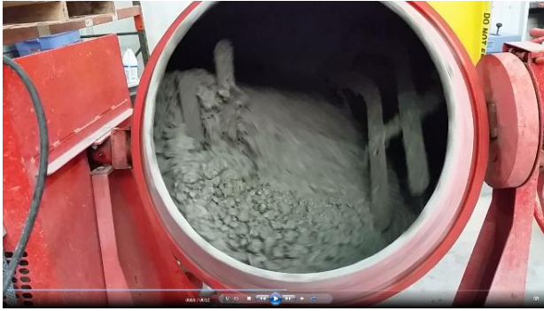
(i) Concrete mixing
