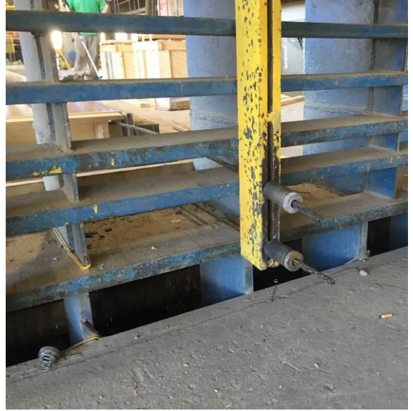
Figure 3.14. Formwork, welded-wire fabric, and prestressing
