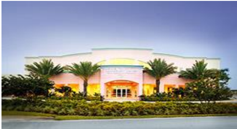
Figure 1. FDOT District Six's SunGuide Transportation Management Center (TMC)
