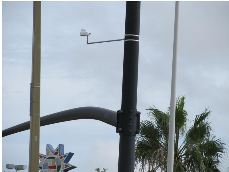
TSP GPS antenna at Fun Spot in Orlando, Florida, photo credit: Frank Consoli, City of Orlando
